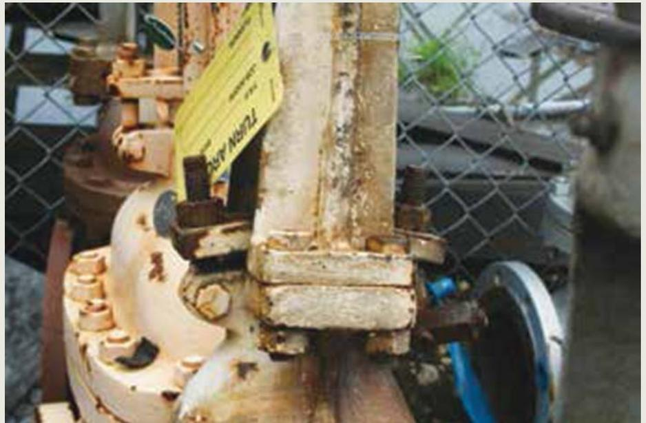
Image 2. An example of a valve that should be replaced.
